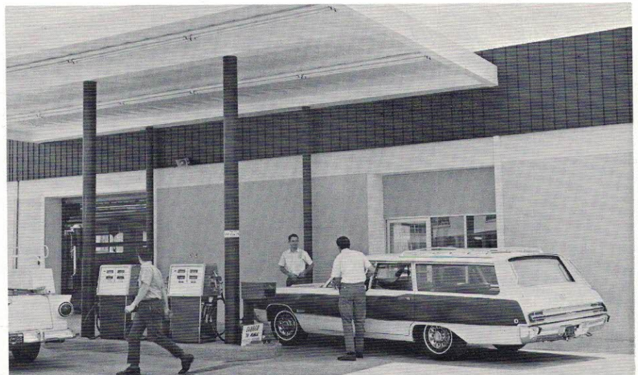
Fueling area for new Transportation Dept.
